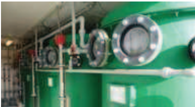
Fixed bed digesters (press fluid)
