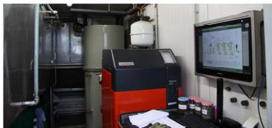
Biogas burner and system control
